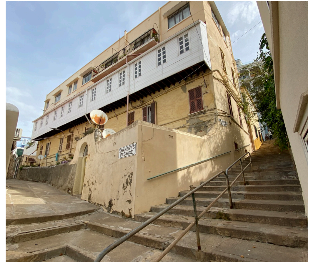
View of the site from the south west corner
